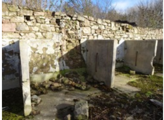
Pigsty divided into bays by concrete structures.
