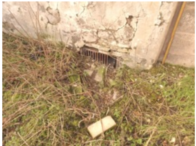
Surface water outlet to north end of site, internal view
