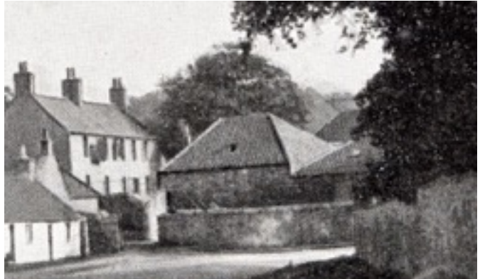
Historical image of the Farmhouse with Chapel (centre) and outbuildings still with roof
