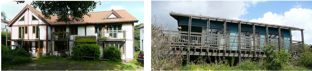
Figure 9: Buildings created with the self-build Segal construction method
